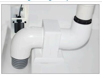
**3.** Willy Vac: using #14 x  $1\frac{1}{2}$ " screws, screw down the Willy Vac to the deck.
